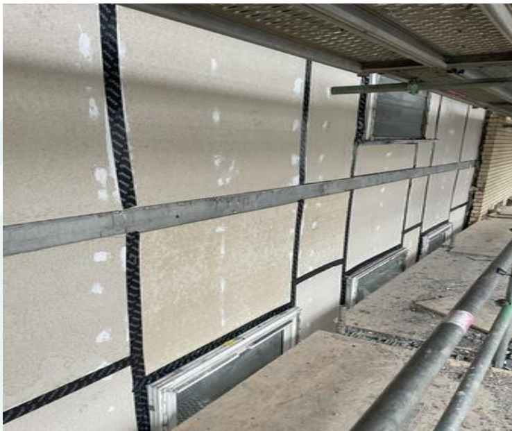
Phase 2 Y wall panels
